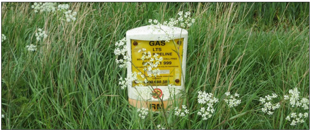
Photo 8. Sign indicating a high-pressure gas main within Field 29, viewed from the south
